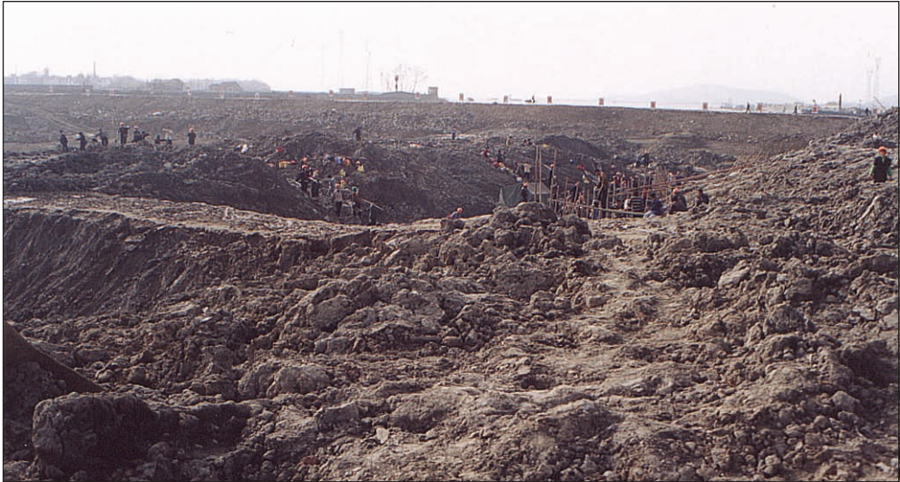
Fig. 2 Government-mobilized workforce rebuilding the dam across outflow of Lake Chao in northern Anhui province. The lake itself lies on the far side of the causeway that forms the righthand half of the quasi-horizon. Photo: Mark ELVIN 2003
