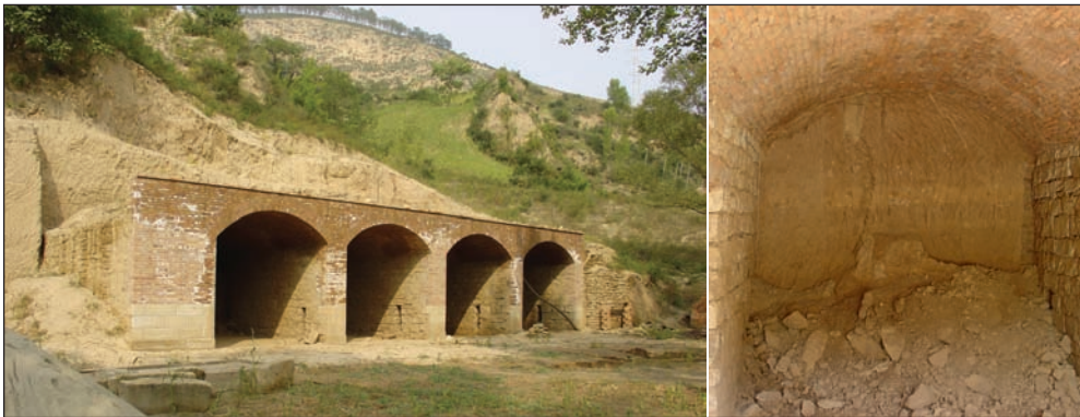
Fig. 11 Different stages of house construction on the Chinese Loess Plateau (Yangjuangou, Shaanxi Province; China). Photos: C. DAHLKE
