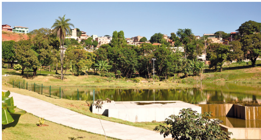
Figure 4: Belo Horizonte, Brazil. Revitalization of urban space with storm and rainwater harvesting parks, example of multifunctional spaces using ecosystem services for increasing social and environmental security of poor districts.
