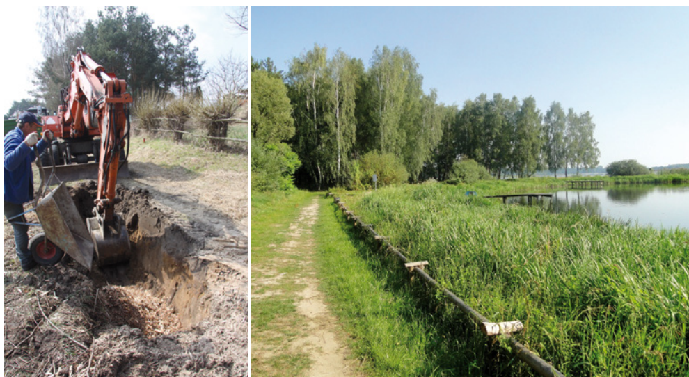
Figure 3: Sulejowski Reservoir, Poland. Restoration of plant riparian zone for buffering the non-point source pollution from agricultural land, combined with establishing of denitrification wall under the road, action funded by EU Project Life+ EKOROB.
